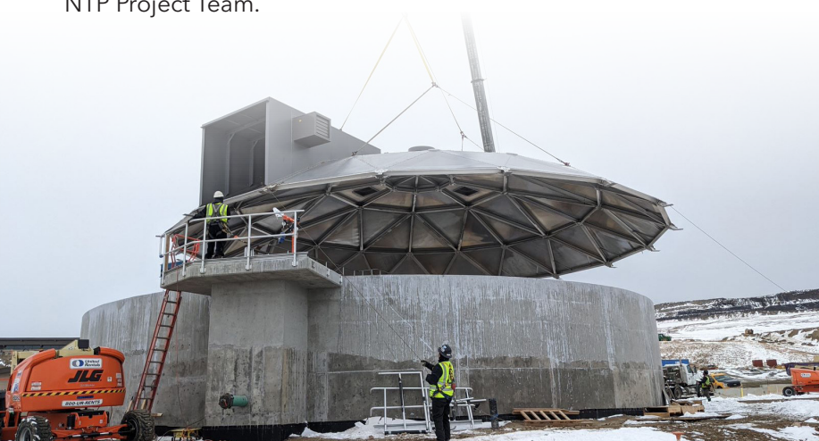
Gravity Thickener Dome Installation
