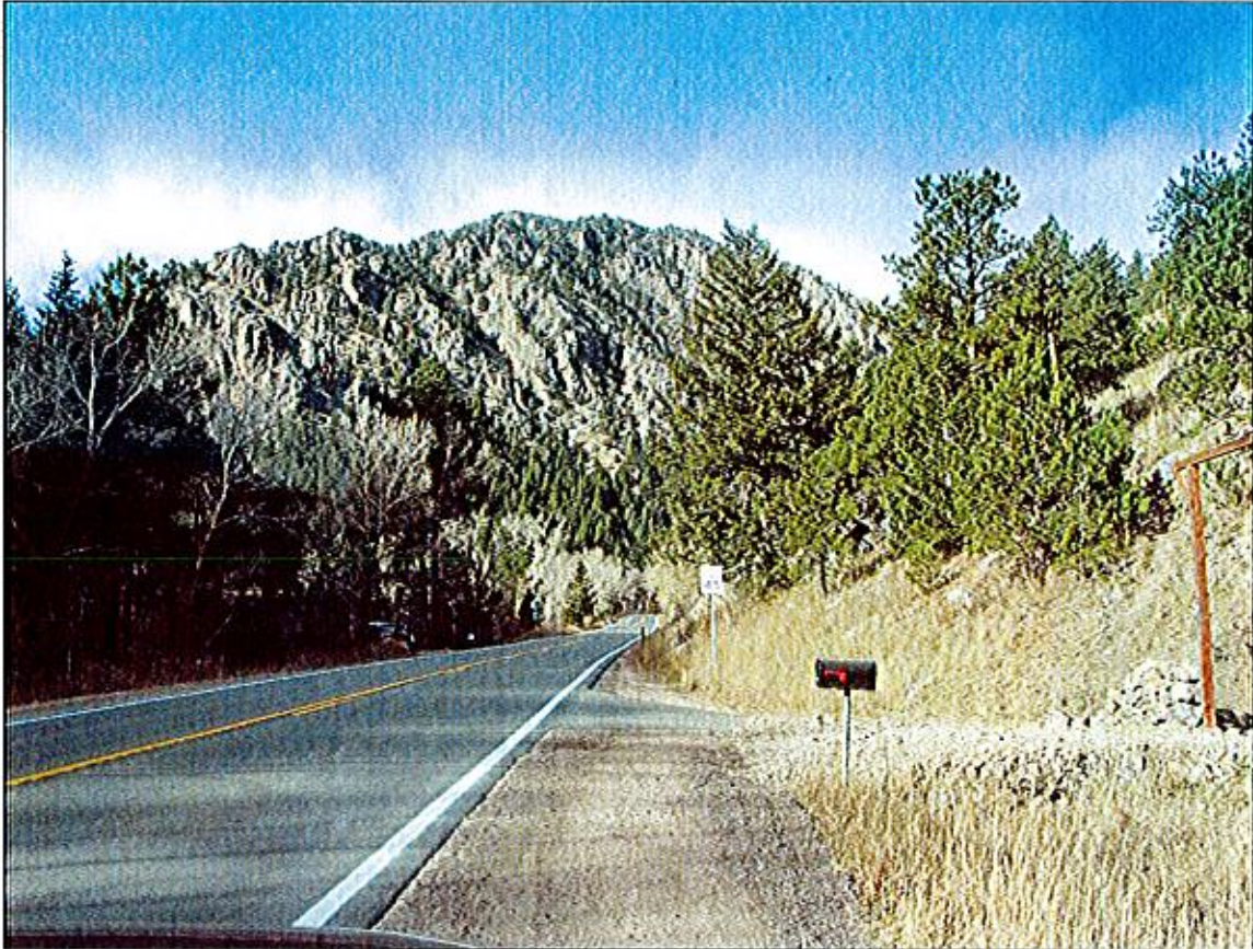
Photo 5 – MP 15.1 Typical cut section / existing pull off
