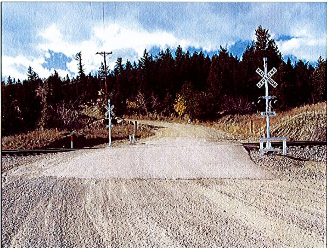
Photo 14 – MP 1.5 Gross Dam Road crossing UPRR (Crescent Siding MP 31.35)
