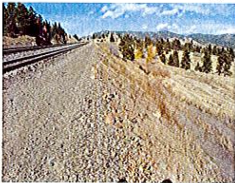
The maintenance road and embankment that parallels the house track.
