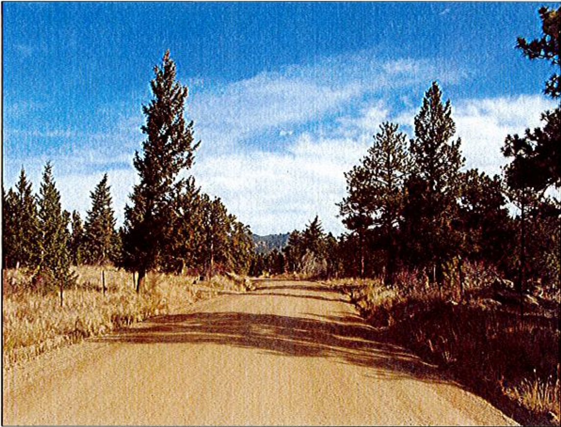
Photo 13 – MP 1.1 Typical Gross Dam Road section
