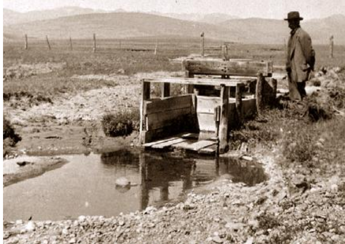
This 1915 photo shows a caretaker standing at the head gate for a ditch flowing into Antero Reservoir.
